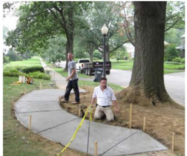
Figure 3. Sidewalk rerouted to increase the distance from the trunk and avoid root damage.
