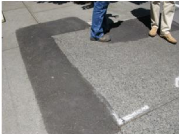
Figure 2. Asphalt ramps/wedge installed to reduce tripping hazards.
