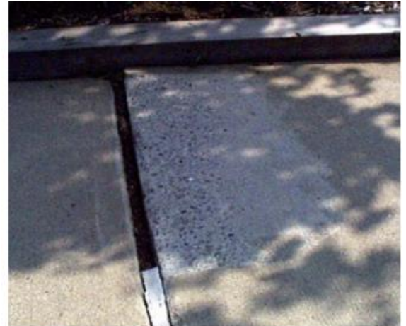
Figure 1. Concrete shaved/ground smooth.
