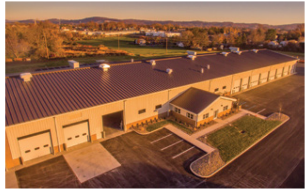
Palmer Township Public Works / Utilities Building
