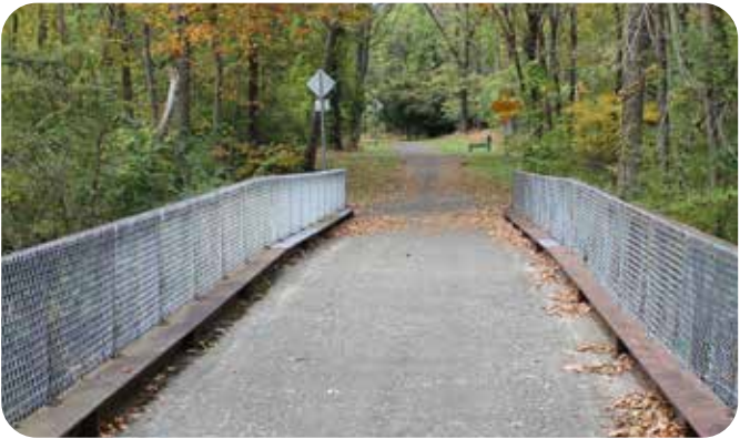
Increase railing height to 42"
